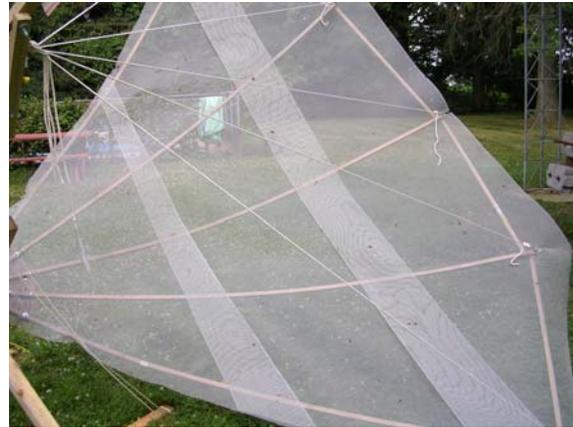
**Fig. 9 - Aluminum screening is tie to the spokes using wire**
