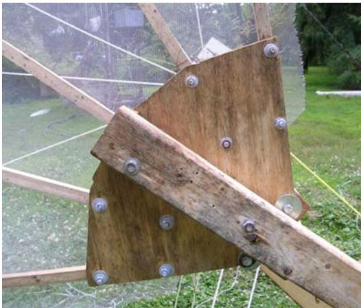
**Fig. 5 - The *spokes* are attached to a plywood center hub with two bolts.**
